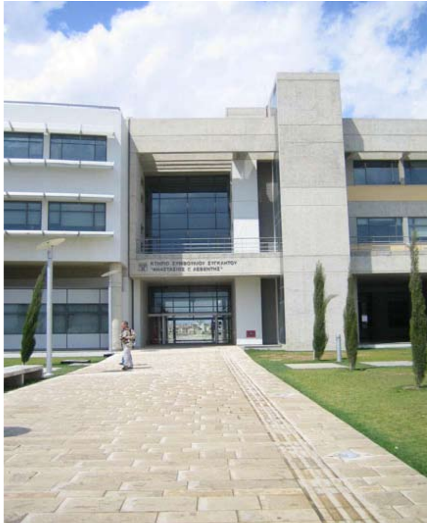
The North Entrance - through the administration building
